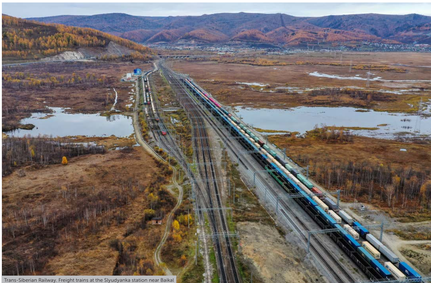
Trans-Siberian Railway. Freight trains at the Slyudyanka station near Baikal
